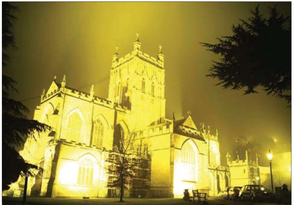
1: An example of poor church lighting in Malvern, illustrating sky glow, glare and the effects of light waste shining uselessly into space. (C Baddiley, taken from CfDS Image Library)
